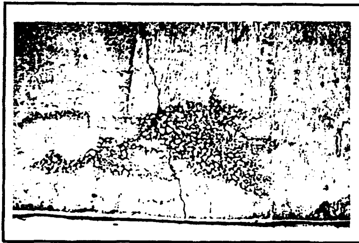
Figure 2.13 Surface Honeycombing (Reference 3)
